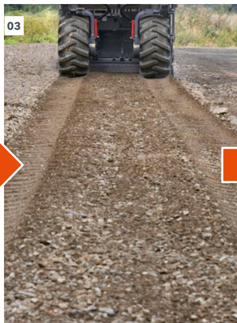
03 Crushing and mixing result: assess and if necessary adjust the parameters
