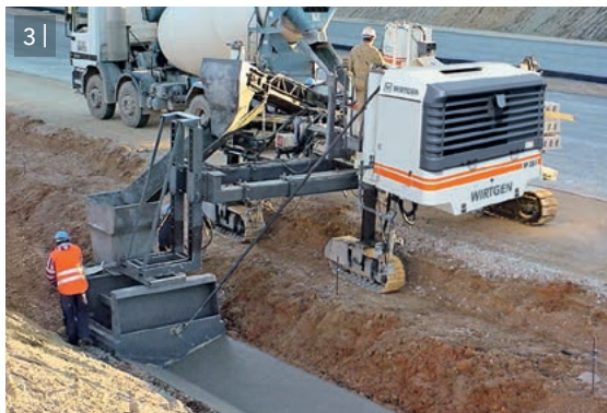
2 | Paving a concrete safety barrier as central reservation.
