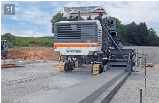
4 | Paving a 8 ft 2 in (3.65 m) wide bicycle path.
