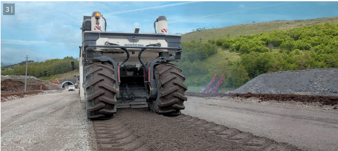
2-3 | Recycled, homogeneous asphalt mix behind the cold recycler.
