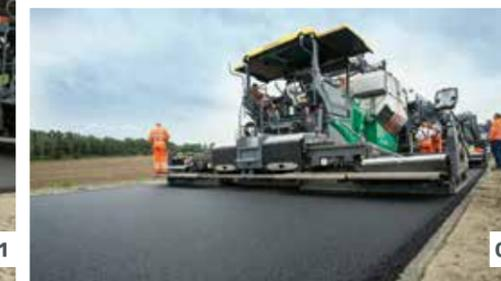
**01** An extra material hopper holding 25 tonnes stores a large quantity of surface course mix.
