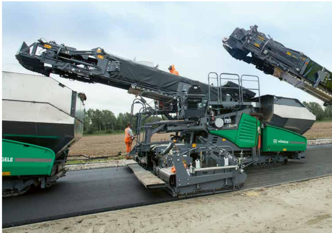
This kind of surface is waterproof, thus protecting the binder course from adverse influences. The high degree of density in conjunction with the layer thickness of 2 to 2.5 cm increases the pavement's resistance to deformation under the influence of heat to such an extent that rutting is massively counteracted, particularly during the summer months.
